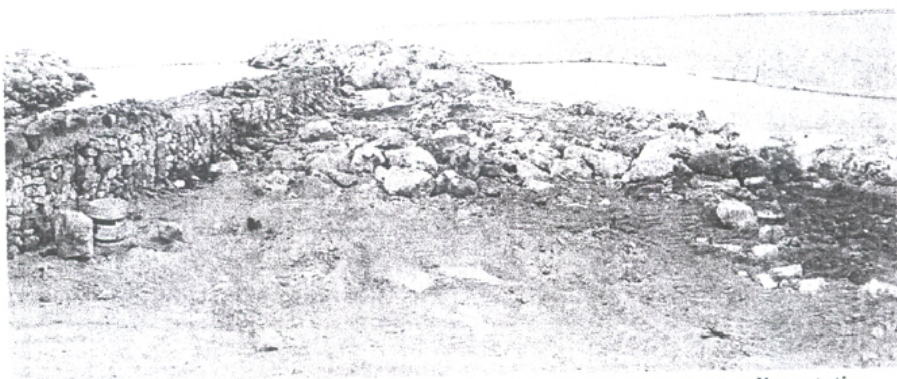
Photo 14: Groyne being realigned. Silt screen in place to prevent excess sedimentation
