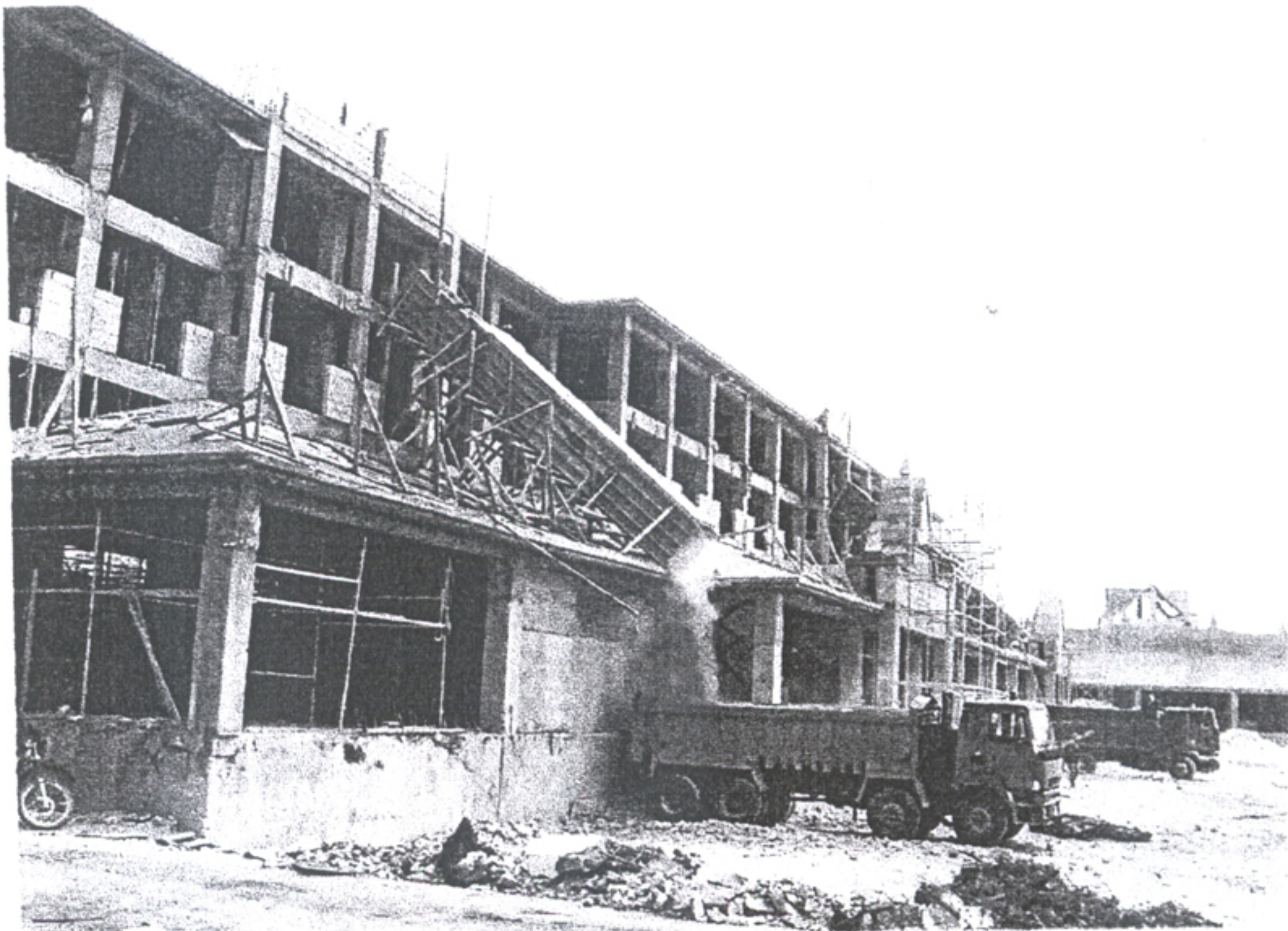
Photo 4: Trucks receiving debris from room demolition
